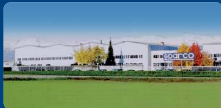
Sparco Headquarter - Italy
